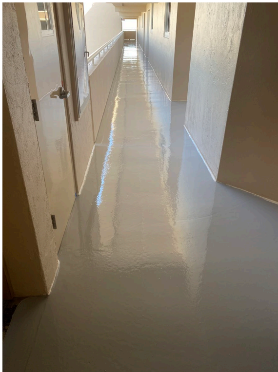
Picture 2: 6 th floor walkway deck coating
